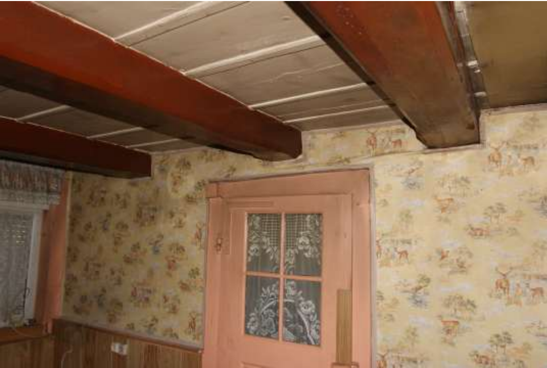
Figure 71. Solivage de la Stube
